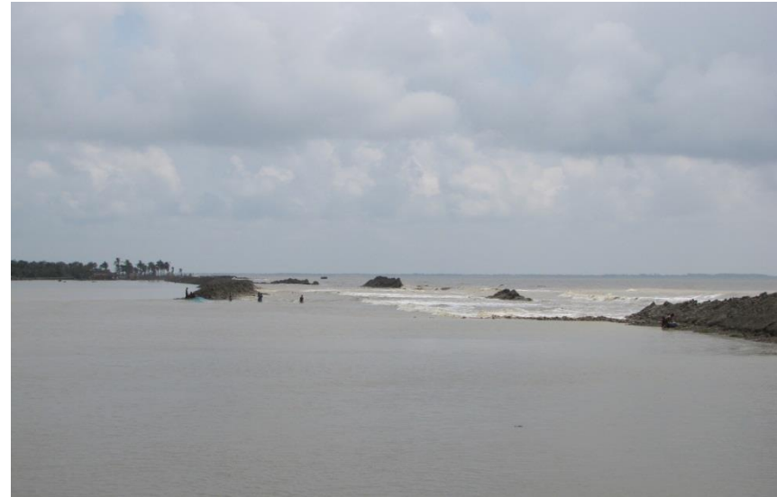
Inundation during high tide
