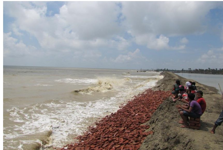
People took shelter above embankment
